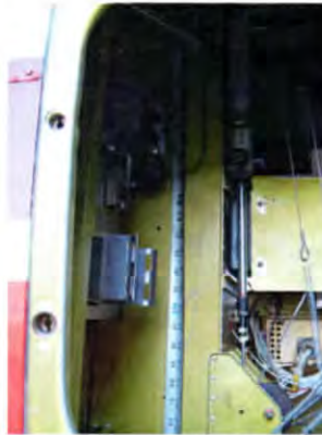
Showing mount installed from left tail access
